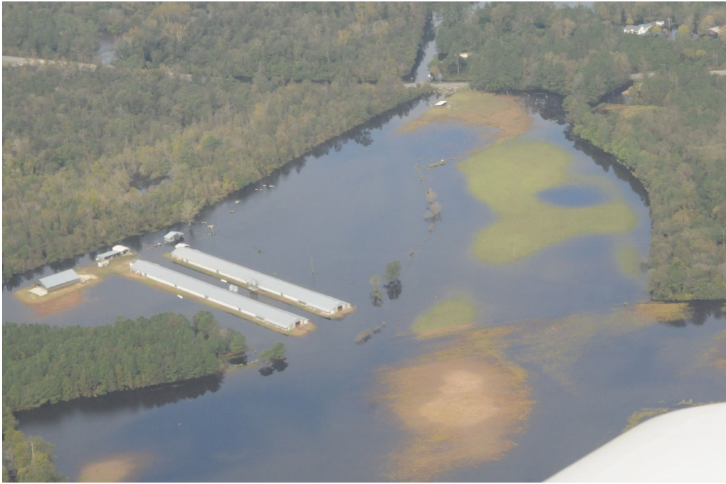
Photo 4. CAFO, Hurricane Matthew Flooding 2016 (image credit CFRW)
