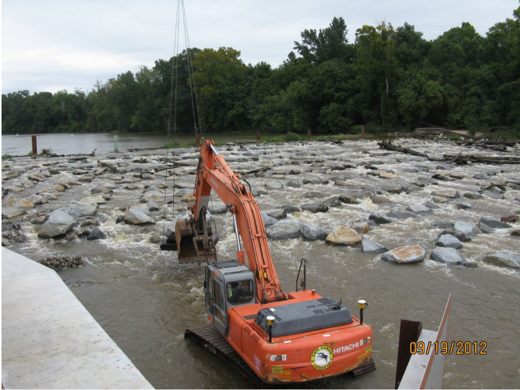
Photo 3. Rock Arch Rapids at Lock and Dam #1 (image credit CFRW)
