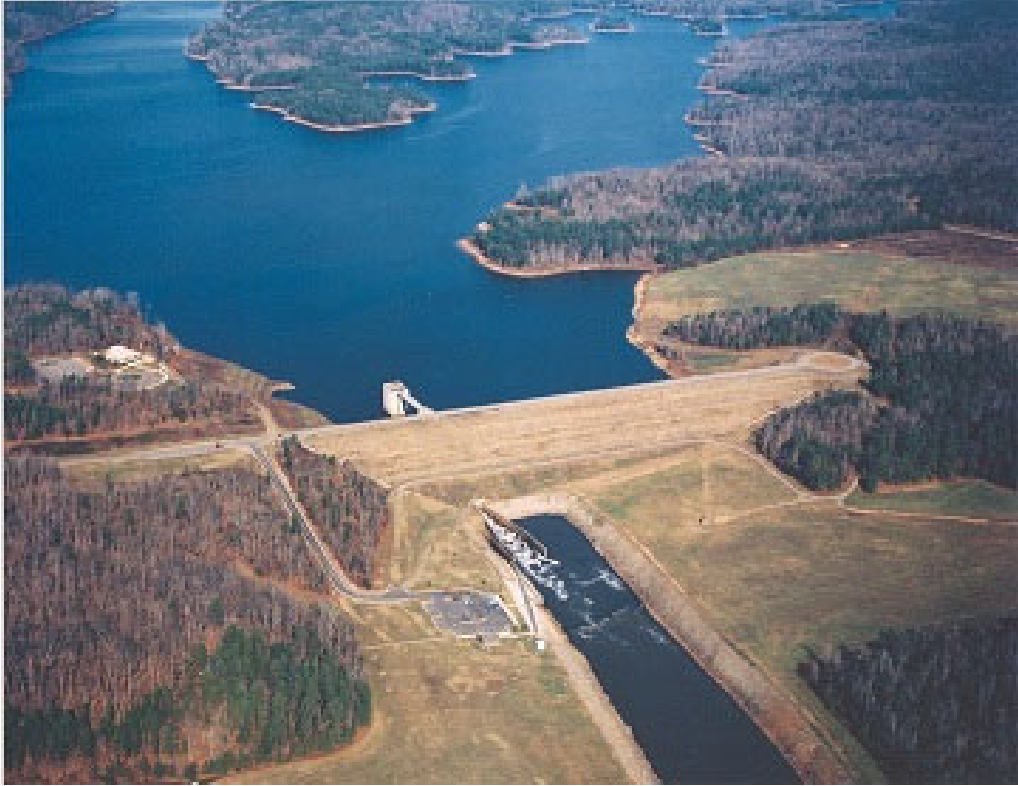
Photo 1. B. Everett Jordan Lake, Dam and Tailrace (image credit USACE)
