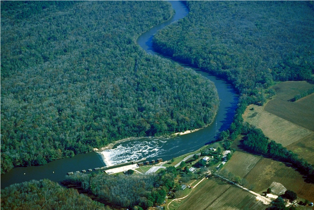
Photo 2. Lock and Dam #1, Cape Fear River (image credit USACE)
